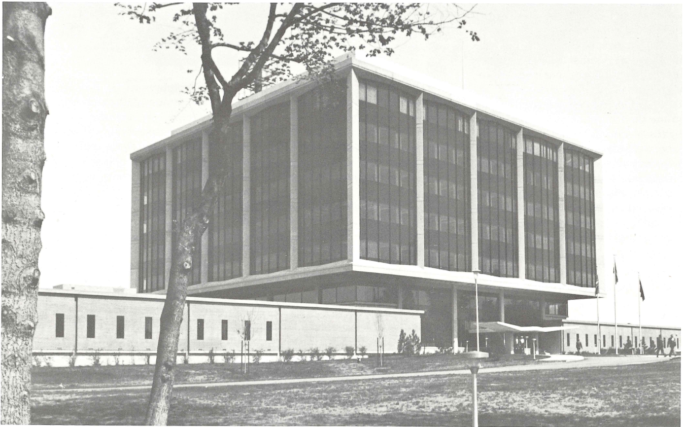
The Sanders Associates facility, Nashua, New Hampshire, that houses the Corporate Computer Science Division.
